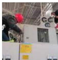
Installation Repair and Maintenance Air Cooling Unit
