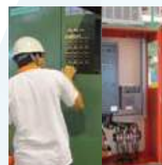
Installation Control Panel Box with PLC, Inverters, Touch Screen, and Servo Motors
